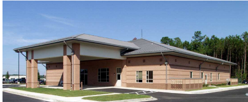
Porte Cochere at Test Administration Area
