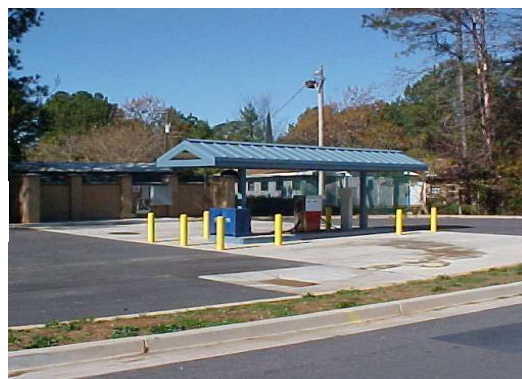
Bus Fueling Station
