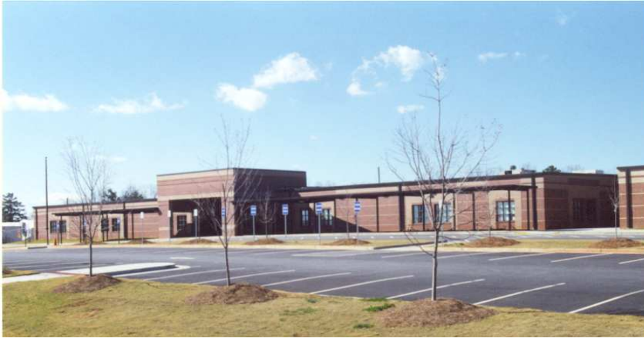
Entrance and Bus Canopy
